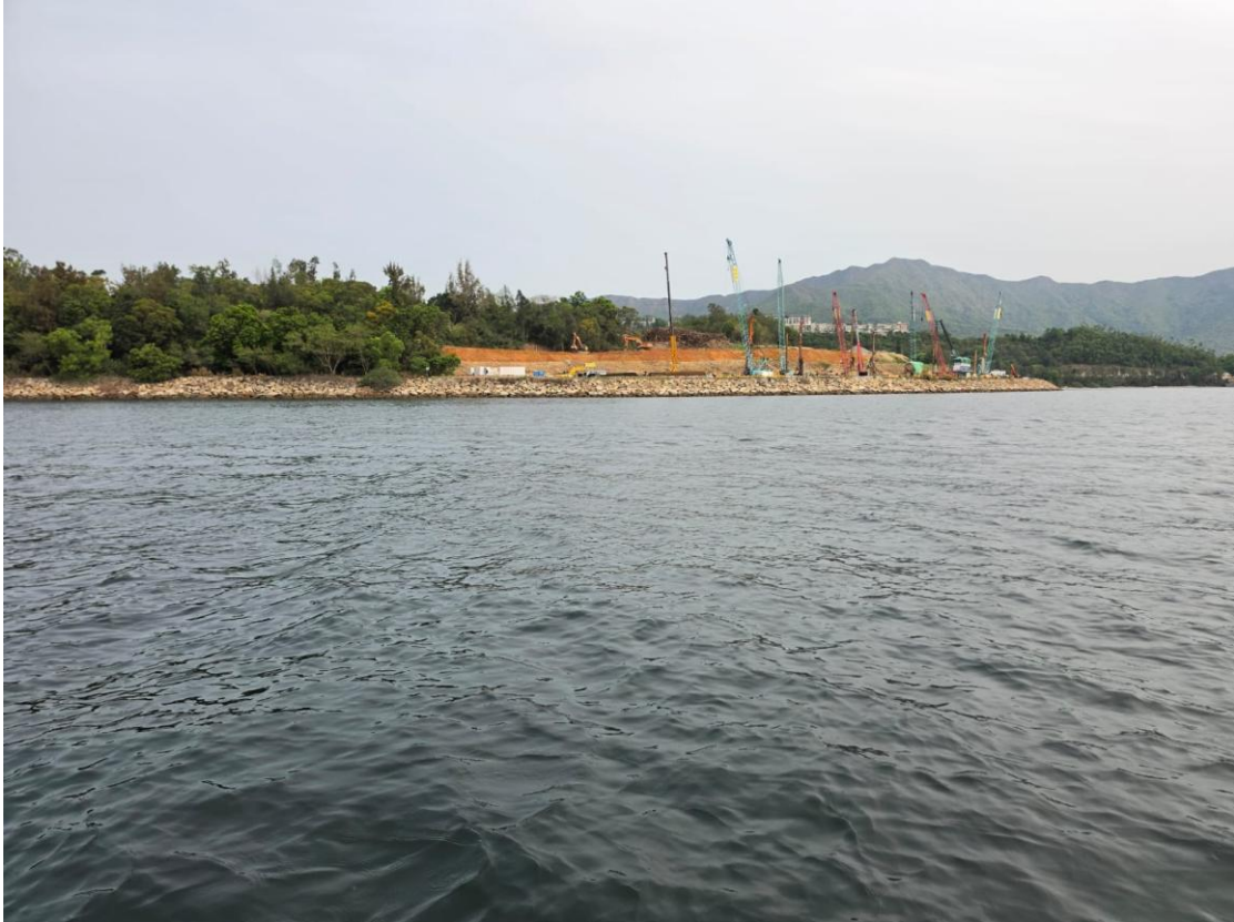
Photos taken by the Environmental Team on 01/04/2026
